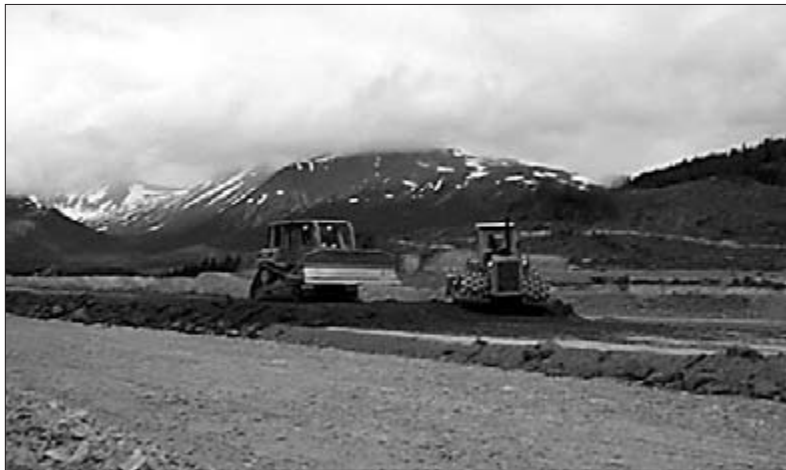
Huckleberry mine near Houston, BC — tailings impoundment construction
