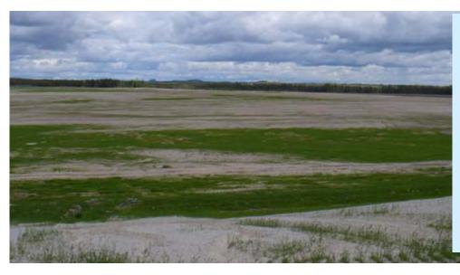
At the abandoned Kamkotia Mine in Ontario tailings that were originally discharged into an impoundment and freely onto the land and are now being rehabilitated using a dry cover. The large area of tailings in this picture is only one of tailings managemen areas. As this site was abandoned Ontario tax payers are covering the \$60-million cost of rehabilitating this site.
