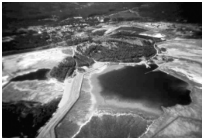
Photo 3. Tailings impoundment at the Sullivan Mine, BC
