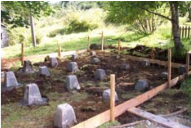
Project area where the traditional medicine facility is being built.
