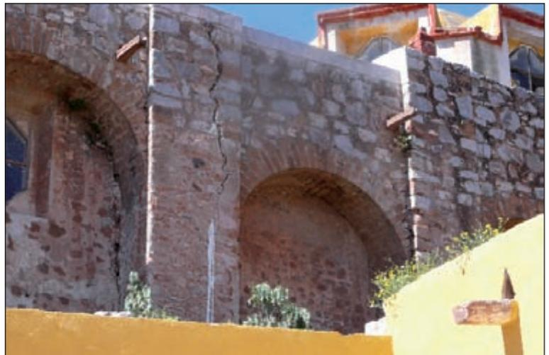
**Evidence of damage already inflicted on a centuries old church, due to vibrations from explosions.**
