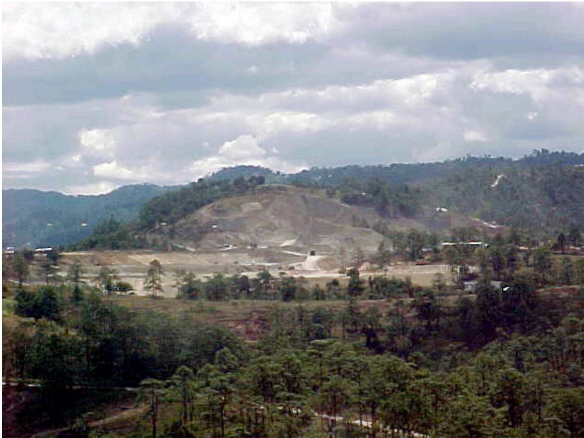
Marlin Mine Facilities Under Construction
