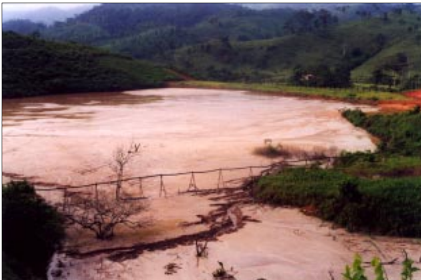
Pipeline carrying cyanide discharge from Hemco Nicaragua's Bonanza mine. Anneli Tolvanen has been working with MiningWatch Canada and the Humboldt Foundation of Nicaragua to document the aftermath of Greenstone Resources' involvement in Bonanza and La Libertad, Nicaragua. (Anneli Tolvanen photo)
