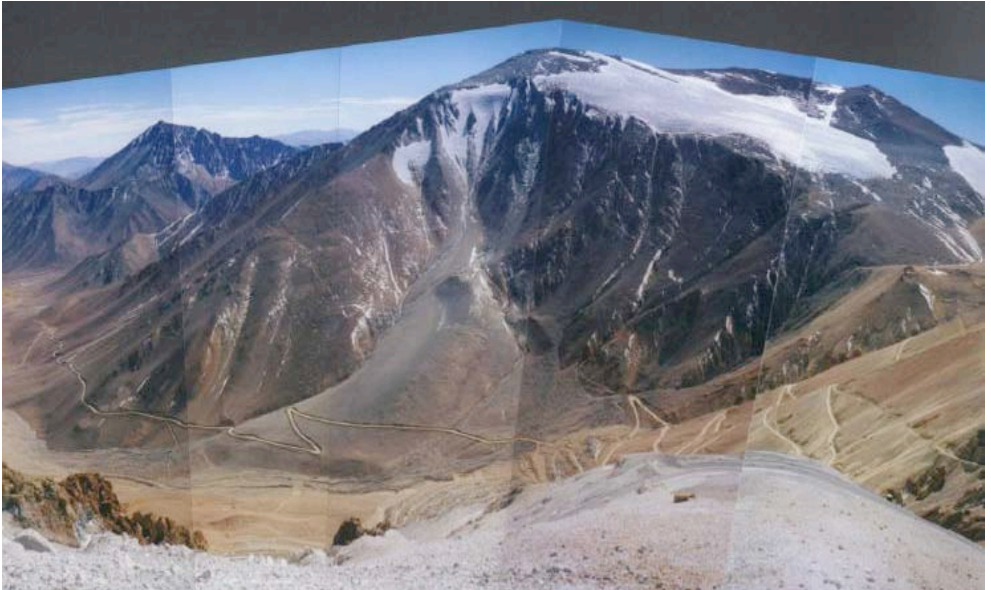
Waste rock disposal site at the headwaters of the Estrecho River (area: 327ha, capacity: 1.274 mt, height: 692m)
