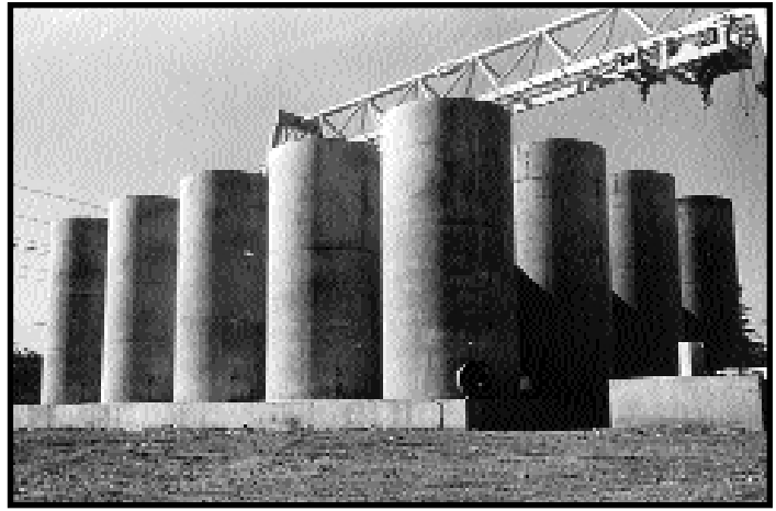
CANDU spent fuel silos.
